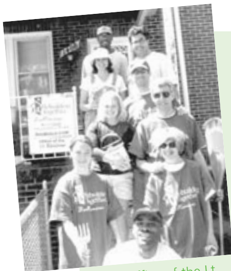
Staff from the Office of the Lt. Governor work on the Butler family house sponsored by B4UBUILD.COM.
